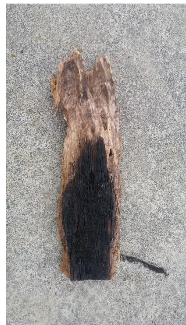
One of the puriri piles photo: B Owen
